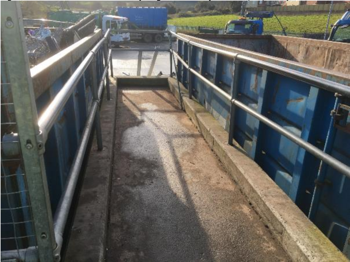
Figure 18: Pedestrian Access to Recycling Containers (E.How 31/02/2019)
