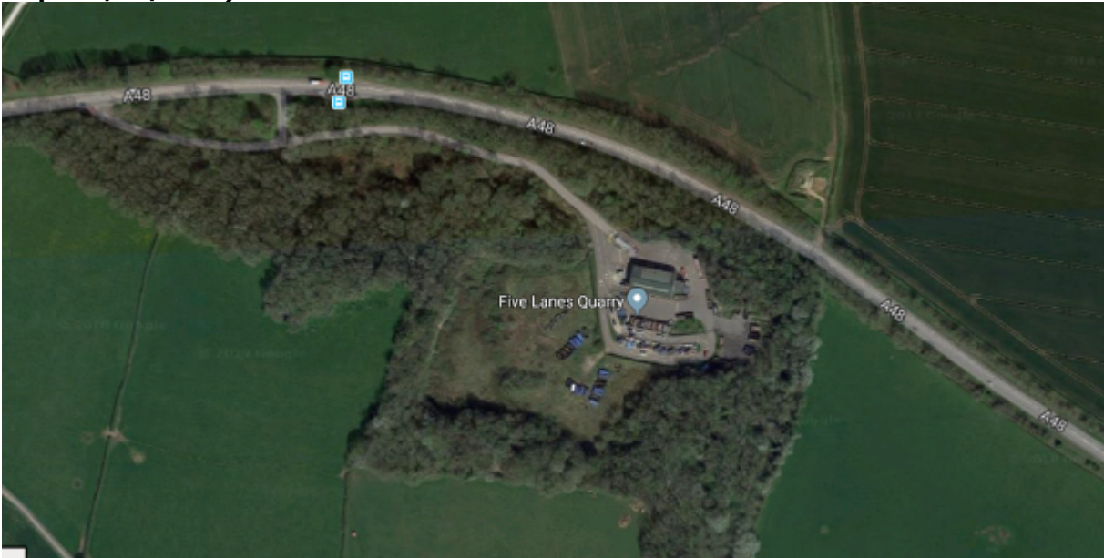
Figure 2: Overview of Five Lane HWRC and WTS Site showing site access road (Google Maps 08/02/2019)
