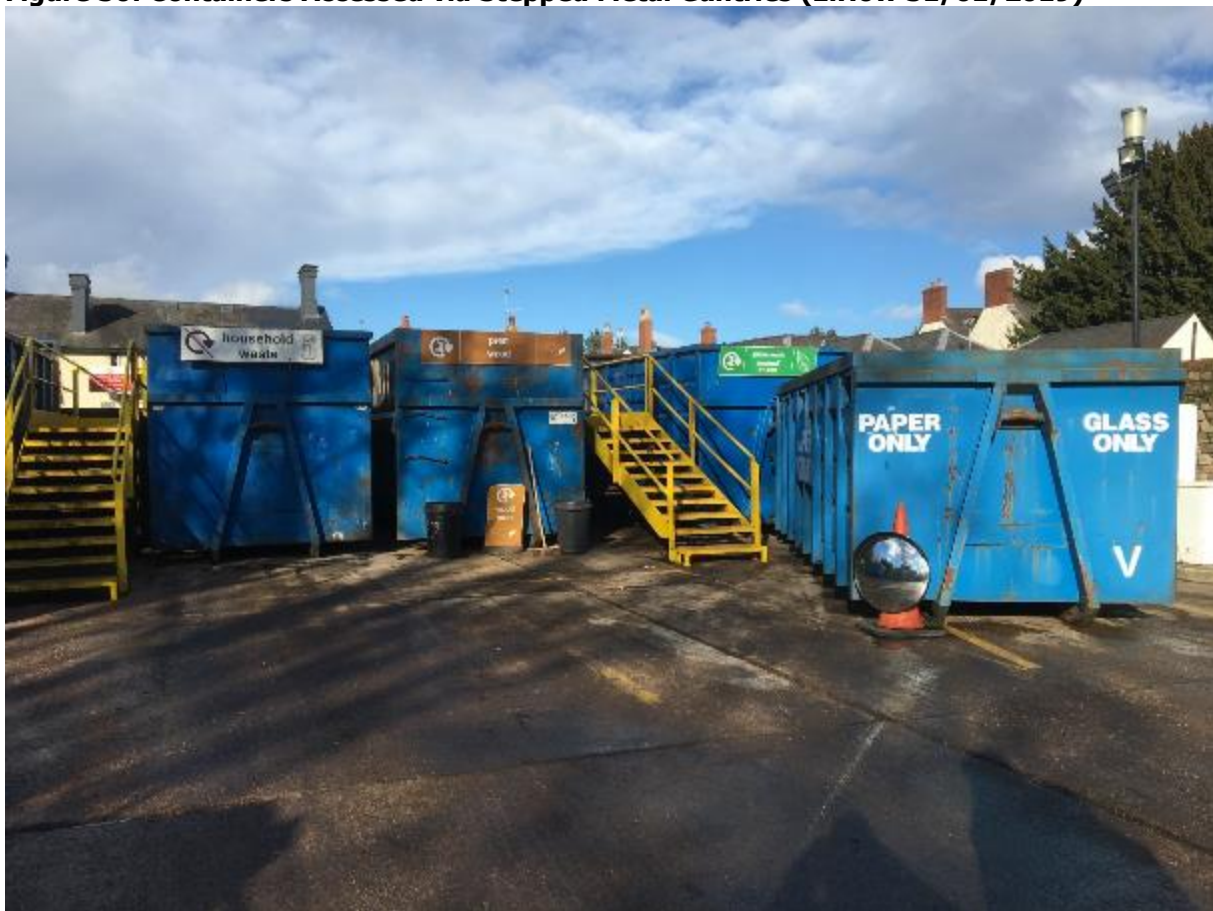
Figure 30: Containers Accessed via Stepped Metal Gantries (E.How 31/01/2019)
